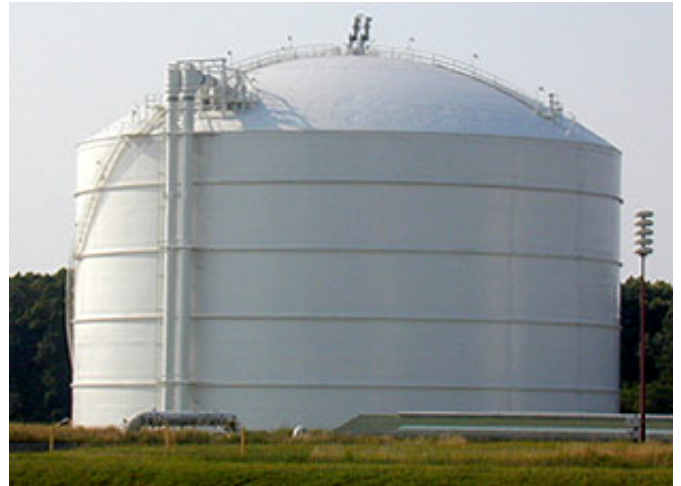
LNG Storage Tank at Cove Point, MD
