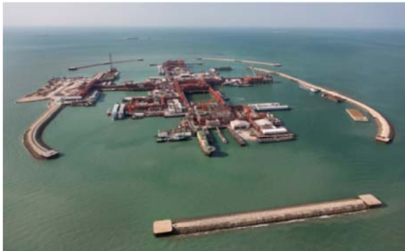
Kashagan offshore facilities
