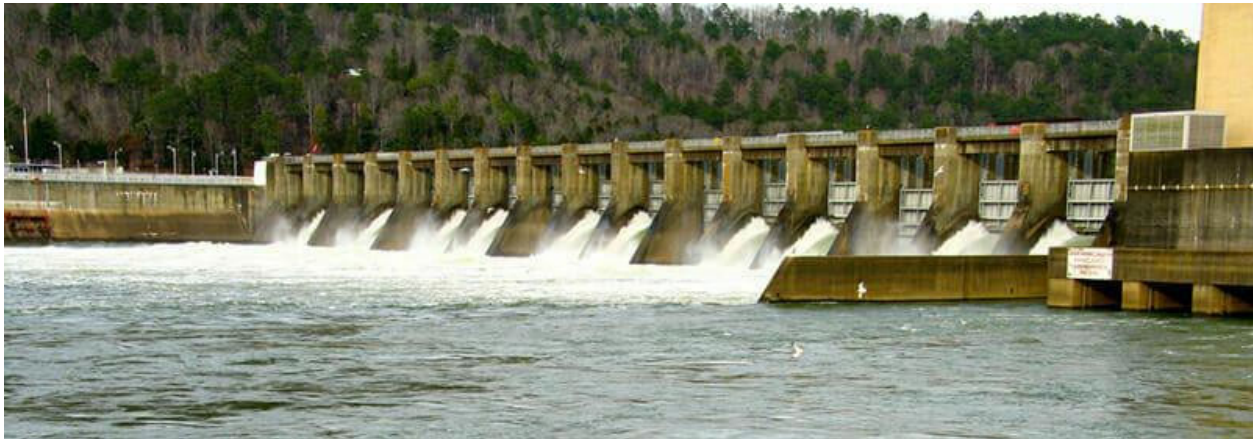
Figure 12-1 — Dam of a Hydroelectric Power Plant
